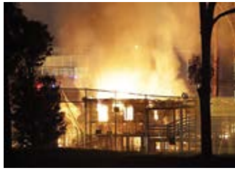
Villawood detention centre on fire.
